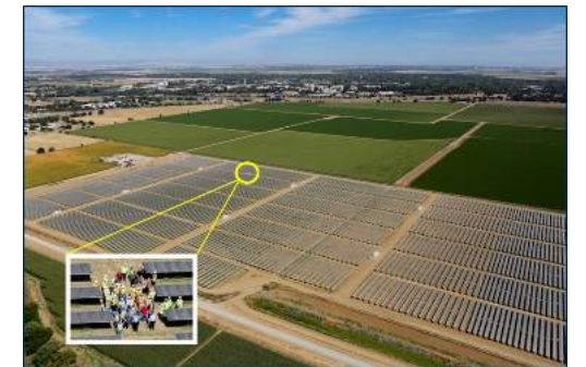
16.3 MW Large Solar Power Plant
