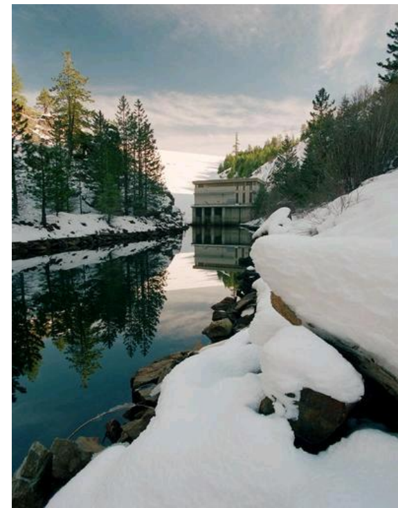
Upper American River Hydro Project – 688 MW
