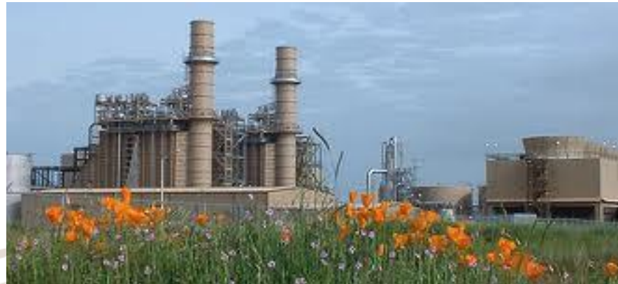
Natural Gas Combined Cycle – 850 MW at 4 locations, NG Peakers 150 MW at 3 loc's
