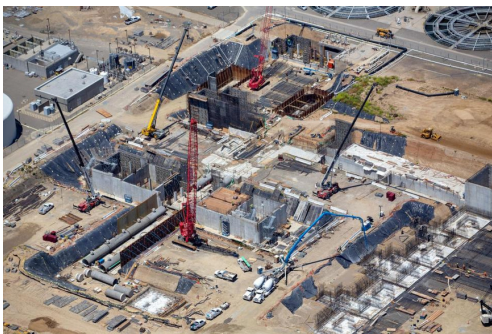
Pictured: Regional San's Tertiary Treatment Facility
